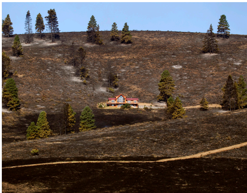
A house near Cle Elum, Washington was able to survive a wildfire on 14 August 2012 as a result of prior removal of trees and brush from the perimeter.”
